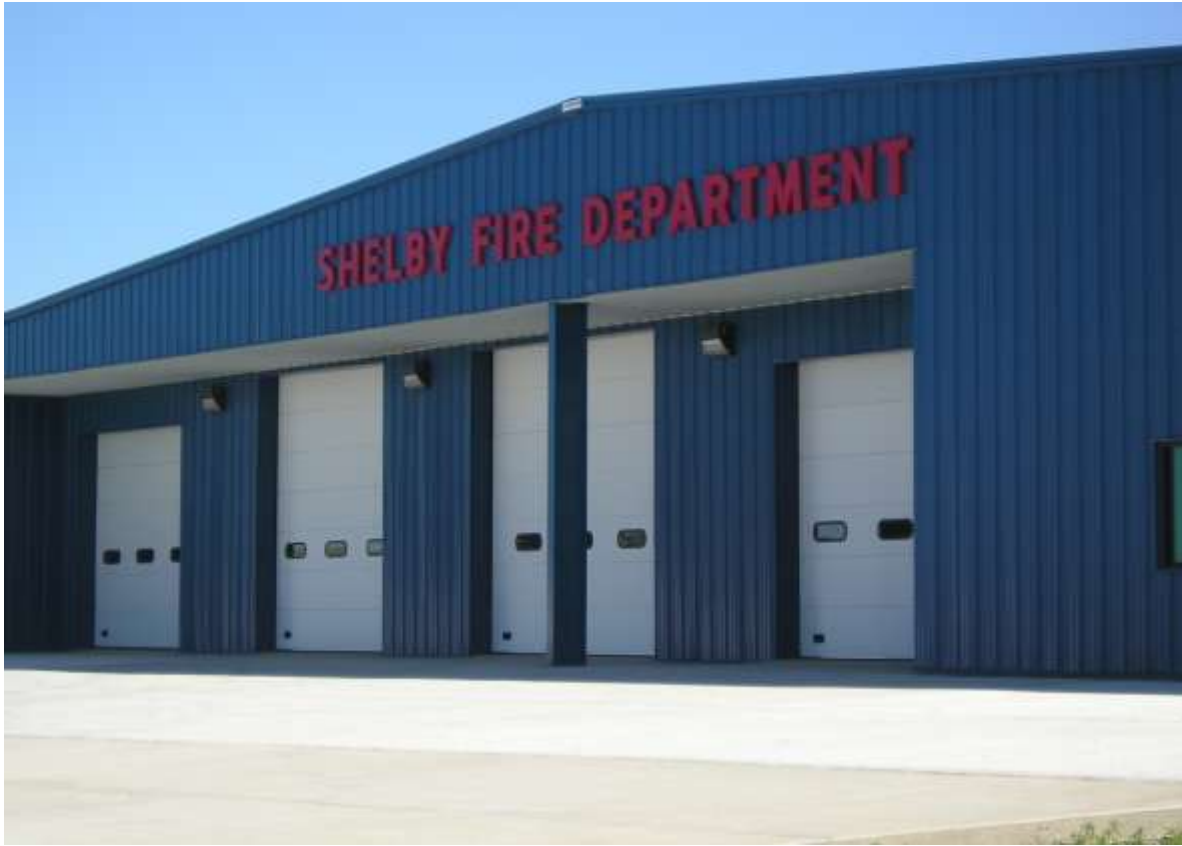
Figure 3.21. New Shelby/South Toole County Fire Department
