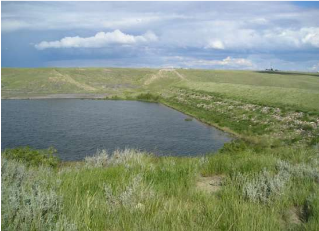
Figure B.4. Shel-oole Dam, West of Shelby
