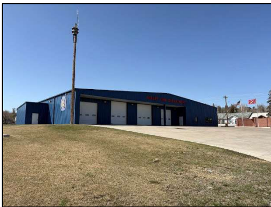
Figure 3 Shelby / South Toole County Fire Dept.
